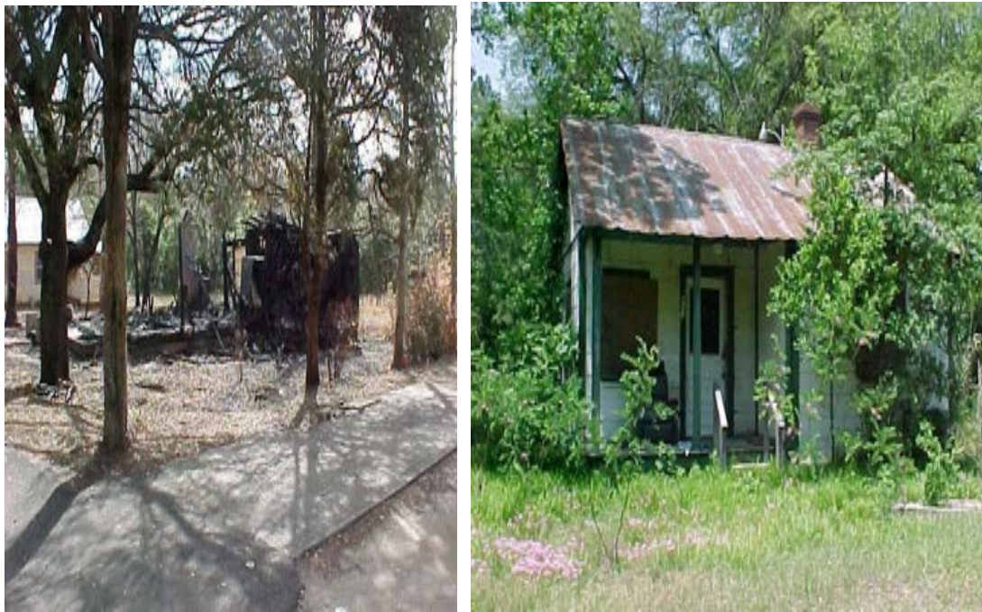
Picture 14. Toole Hill Project – PHASE I – BEFORE
