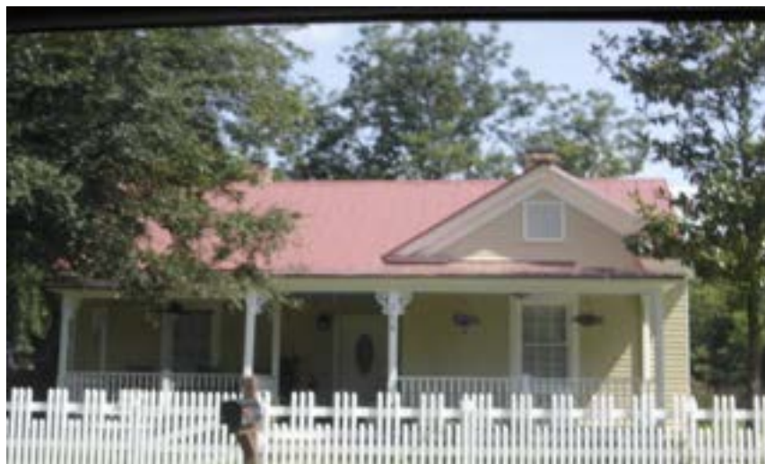
Picture 18. Marion Street Housing Project
