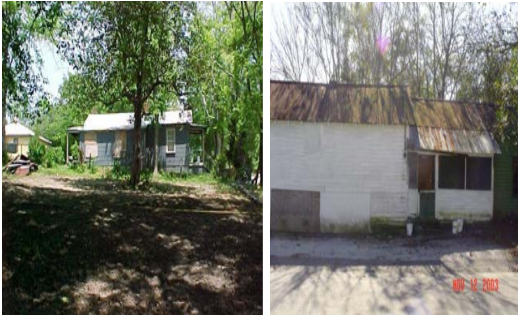
Picture 15. Toole Hill Project – PHASE I – BEFORE
