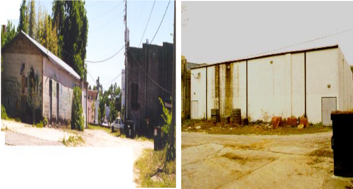
Picture 10. Aiken Corporation Parker Project – BEFORE
