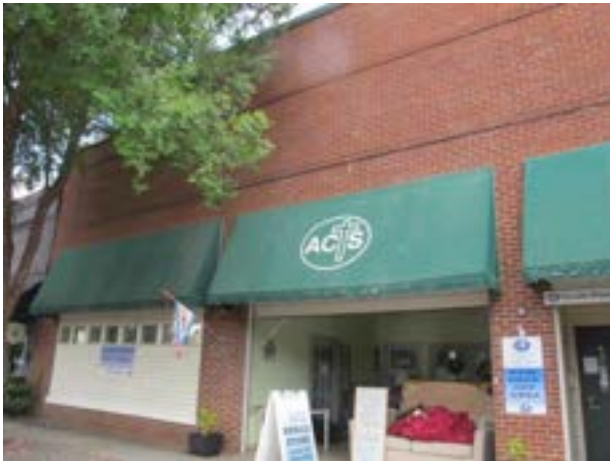
Frontage of site and improvements along Hayne Avenue
