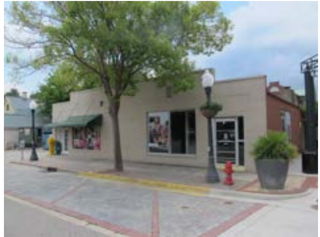
View of existing building along Newberry Street
