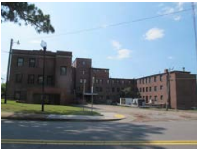
View of existing hospital building on site
