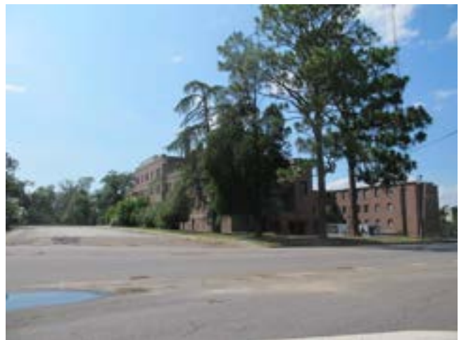
View of existing building and vacant land
