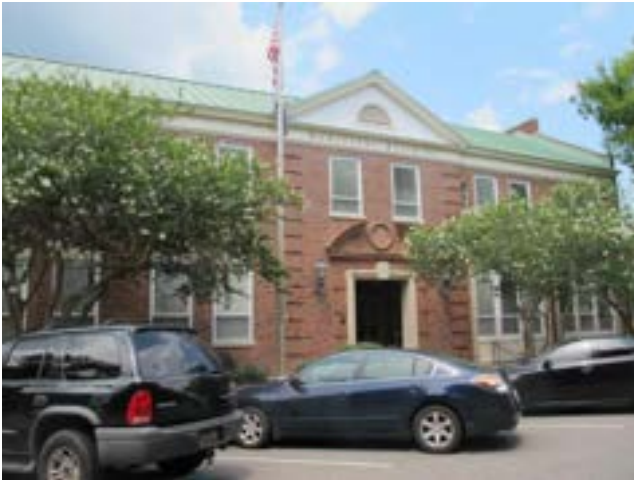
View of existing Municipal Building along Park Avenue
