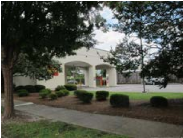
Site frontage along Pendleton Street
